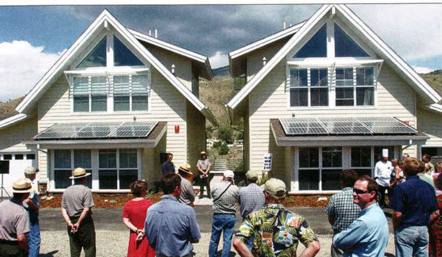
Many sustainable features were incorporated into the Yellowstone homes, including photovoltaic panels, passive solar configurations, and insulating concrete forms. Thicker foam panels were used on the exterior face of the walls to achieve an R-32 rating. PHOTOS: QUAD-LOCK BUILDING SYSTEMS
