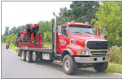
A boy's dream: A big truck, a big hole and lots of concrete and dirt.
